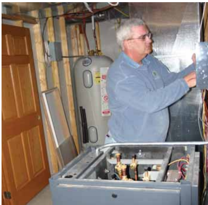
Above: Northern Electric Cooperative Member Service Director Doug Hamilton checks the electrical wiring of the NorAire unit in the Sumption’s home near Frederick, S.D. The foreground of the photo shows the indoor portion of the heat pump (with the top of the unit removed). Behind Hamilton is the home’s air exchanger and Marathon water heater. Top: The Sumptions – Jonathon, 9; mom, Stacy; Hannah, 7; Haley, 11; Jacob, 3, dad, Eric and Maddie, 1 – move into their new home in February. The home will be heated by an innovative air-source heat pump. Opposite: The Sumption’s will move into their new home near Frederick in February. Photos courtesy Tom Green
