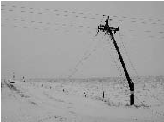
This pole, just east of Larry Smejkal's farm south of Wagner, was one of many that was snapped off just above ground level. Looking down the fenceline, not a pole is standing as far as the horizon.
