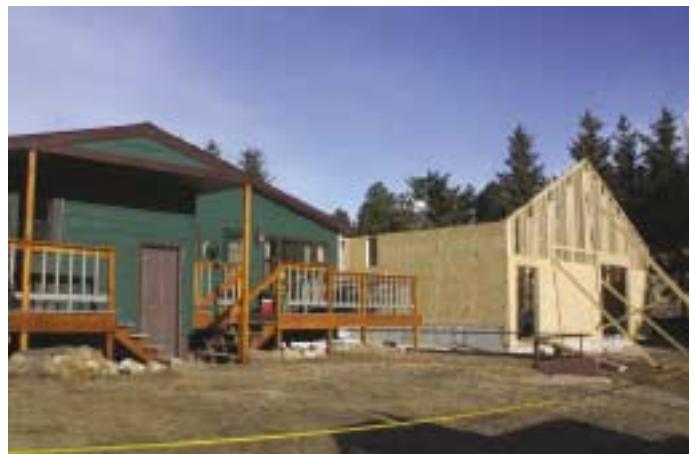
Top and Cover: This seasonal home was recently constructed west of Custer, S.D., on Black Hills Electric Cooperative's lines. Seasonal accounts make up about 19 percent of the cooperative's total accounts and account for 5 percent of the kilowatt hour sales. Left and Above: Black Hills Electric Cooperative Manager of Marketing and Member Services Mike Chase talks with the construction forman at the site of a seasonal home undergoing remodeling with an addition north of Custer.
